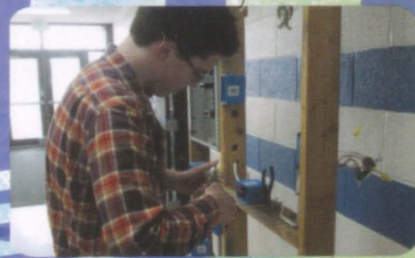
Jordan Johnson putting in an outlet
