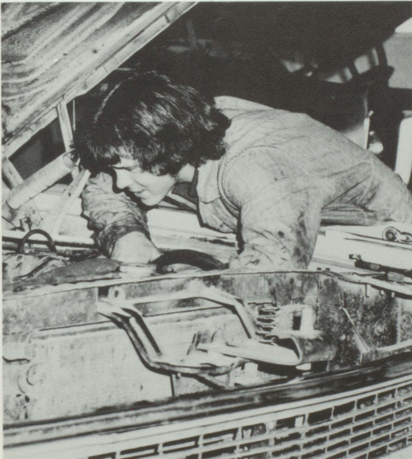
"Oh, well, who needed that bolt anyway?"
