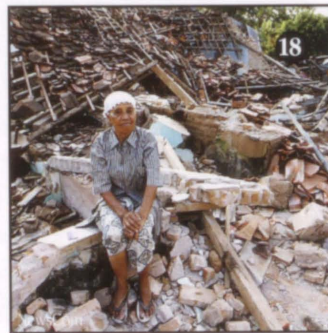
18. A 6.3 magnitude earthquake struck Indonesia on May 27, 2006, killing more than 5,800 and injuring 36,299. Thousands of aftershocks followed and hundreds of thousands were left homeless in central Java.
